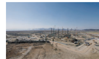
Scene of the construction
