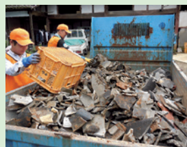
Employees removing rubble at individual homes in Mashikimachi
